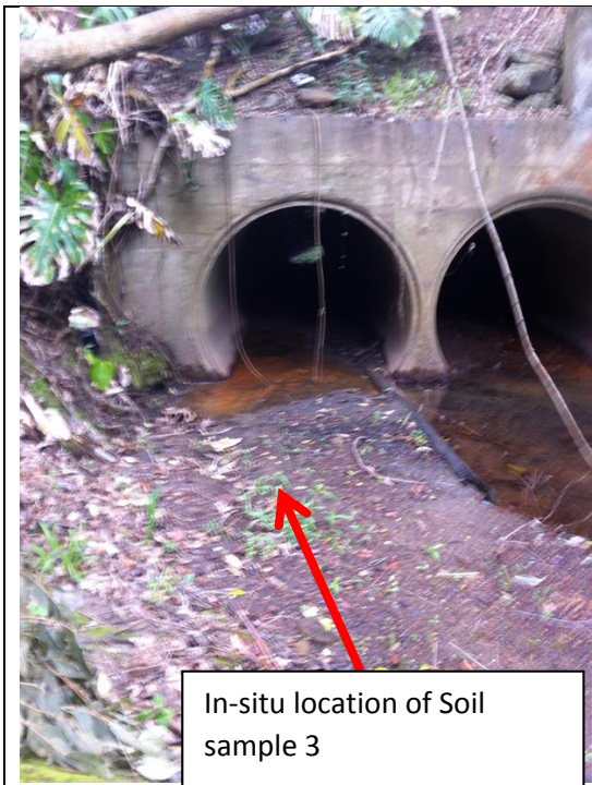
Figure 22: location of sample 3. Note this is the material that will wash into the creek with the next onset of rain
