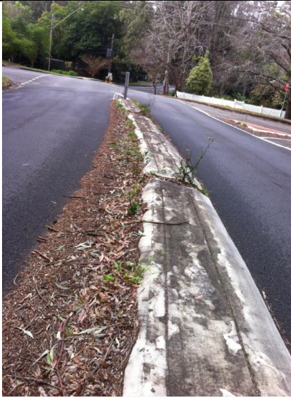
Figure 29: Location of sample 4. Note the presence of live vegetation growing in the material
