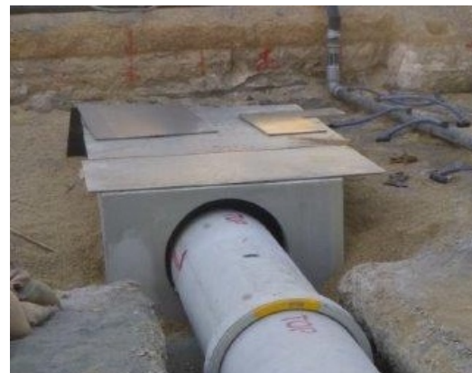
The next day, pipework installed
