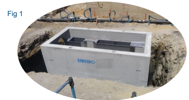
Fig 1 An H90 installed into water charged soil. Substantial savings were generated by minimal site works. The reinforced concrete chamber is installed directly into final position without additional base slabs and tie downs. Risers and cover slab are then added to match final site levels.
